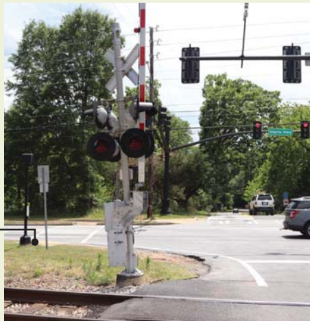
Sidewalk at Atlanta Highway and 6th ends
